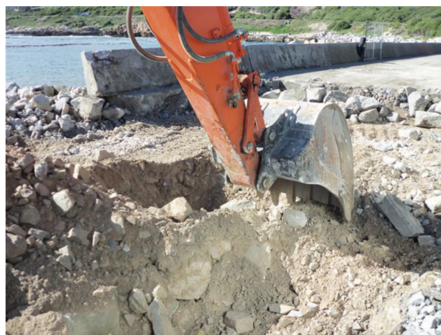
After removal of concrete deck: Test hole at 1 m deep
