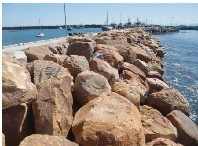
Stage 8: Complete single layer 4-6 t rock
