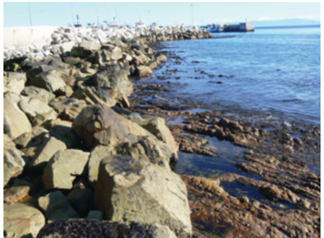
Breakwater founded on rock reef
