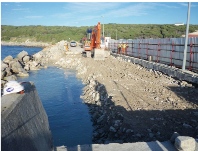
Stage 2: Trimming back existing sand core
