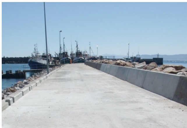
Stage 9: Completed 7 m wide 800 mm deep concrete roadway
