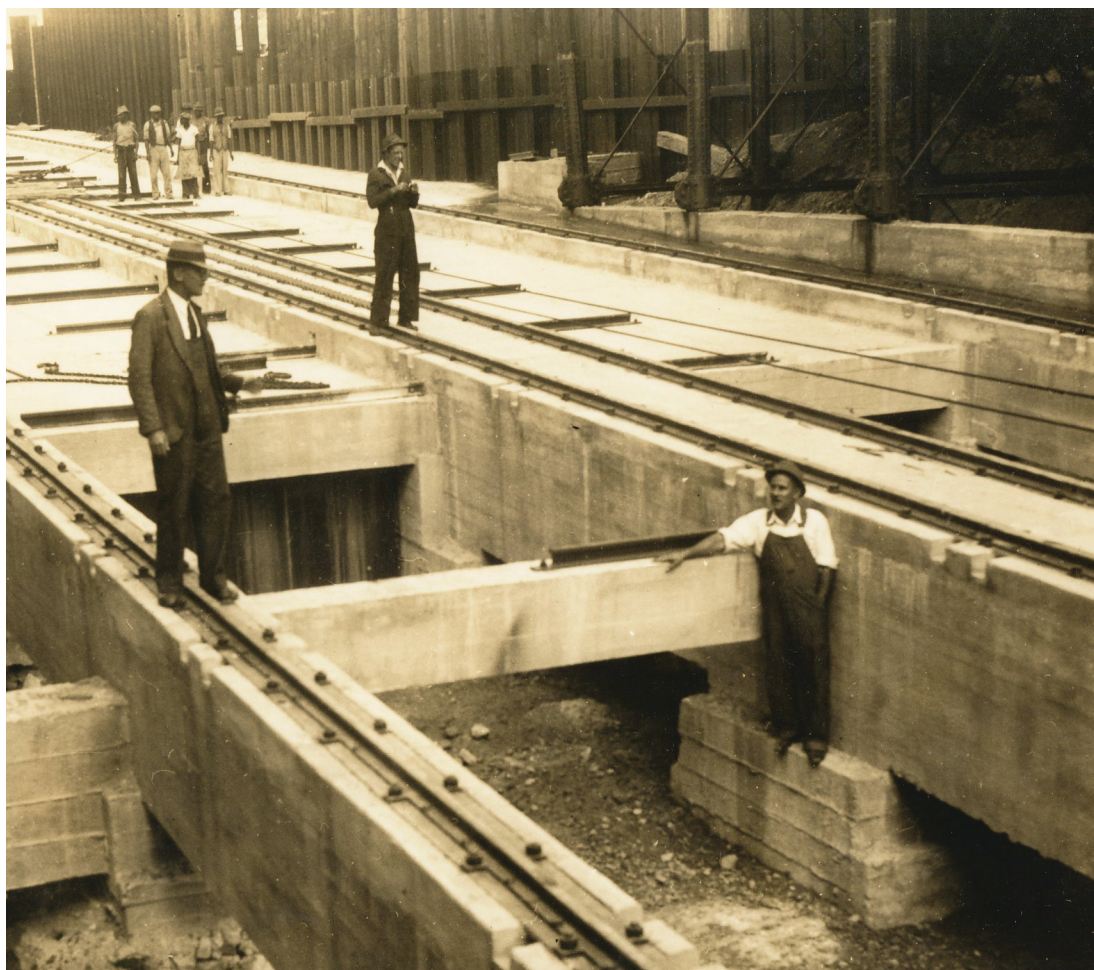
1,200 tonne Henderson Slipway constructed in 1945 to military specifications – still in use as common user facility. An estimate of the load capacity of the keel ways beam, assuming 25 MPa concrete, is sufficient for the keel block loading of a Panamax container ship.
