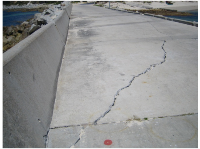
Shear crack running for 30 m along structure length
