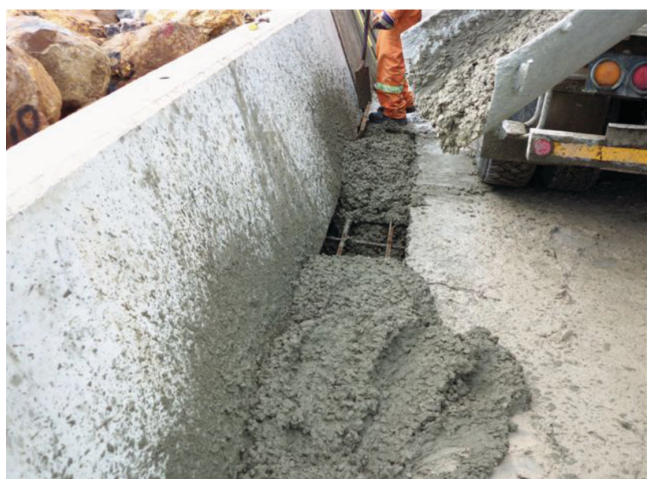
Stage 7: Stitchcast parapet walls to concrete roadway
