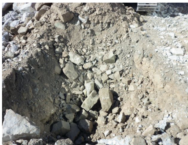
After removal of concrete deck: Test hole at 1.5 m deep
