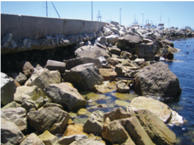
Rock armour defence collapsed
