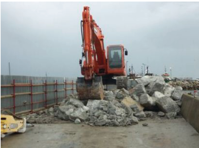
Stage 1: Demolition of existing concrete roadway
