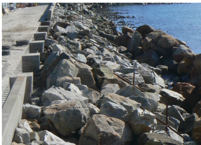
Stage 6: Complete double layer 1-3 t rock
